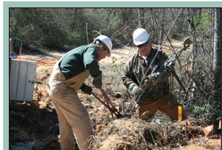
Maintenance: Clarke-Washington EMC linemen Dwight Pugh and James Koen anchor a guy wire from a powerline on Club Wiley Road in Jackson in March. Replacing and securing guy wires to the ground ensures the strength of the power pole and line, while the yellow guy guards notify people of the existing line, watching out for their safety.
