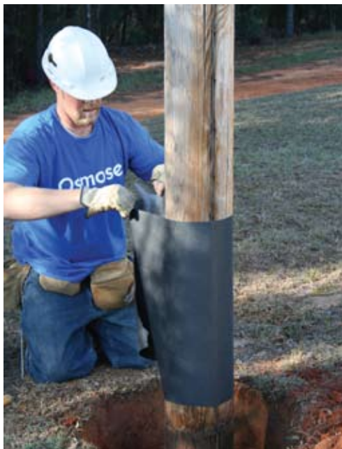
An Osmose crew member wraps a waxy type paper around a treated power pole. Three, two-man crews inspected about 5,000 poles in the areas north and east of Millry in December.
