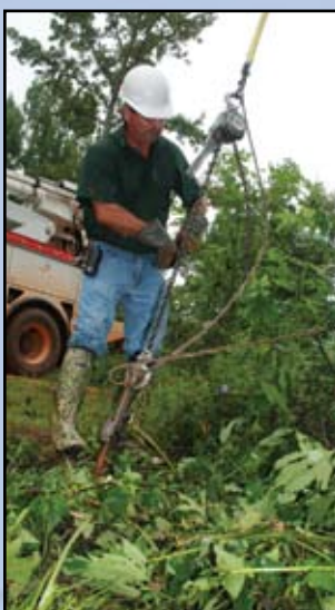
Terry Hooper with CWEMC tightens a guy wire after storms from Hurricane Fay in August.
